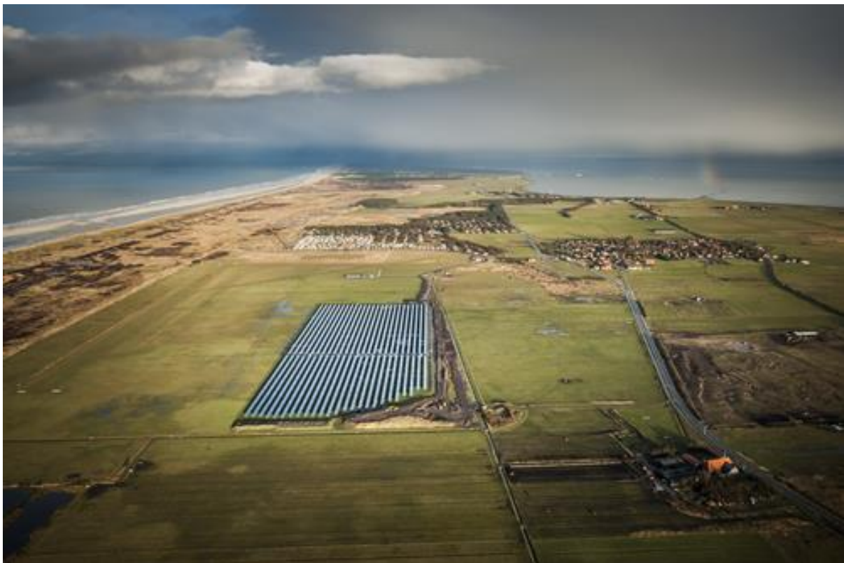
FIGURE 5. THE AMELAND SOLAR FARM 17 .
